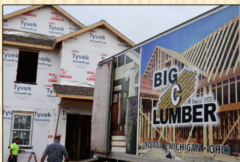
Truck unloading windows into a new construction house.
